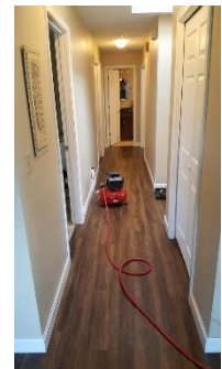
New paint and trim casing
